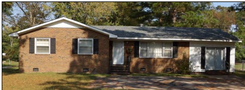
Photo 74: House at 304 W. 16 th Street. Note the wood windows
