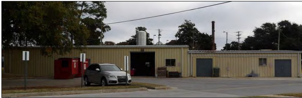
Photo 46: Southwest Elevation of the Machine Shed.
