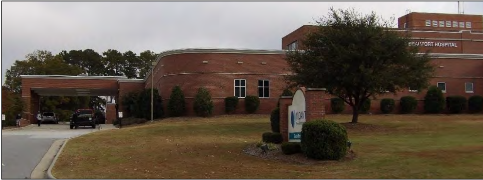
Photo 43: South Elevation of the 2008 Addition.
