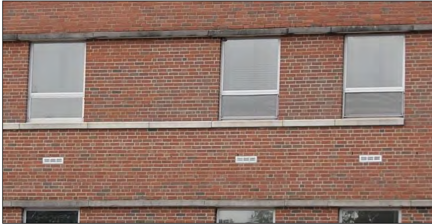
Photo 39: Window Detail on the Eastern Wing.
