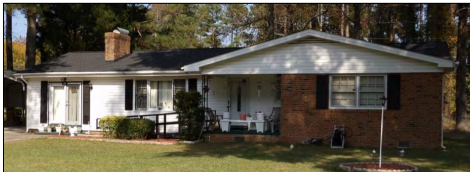
Photo 72 House at 202 W. 16 th Street, example of both brick veneer and vinyl siding covered by a cross-gabled roof.
