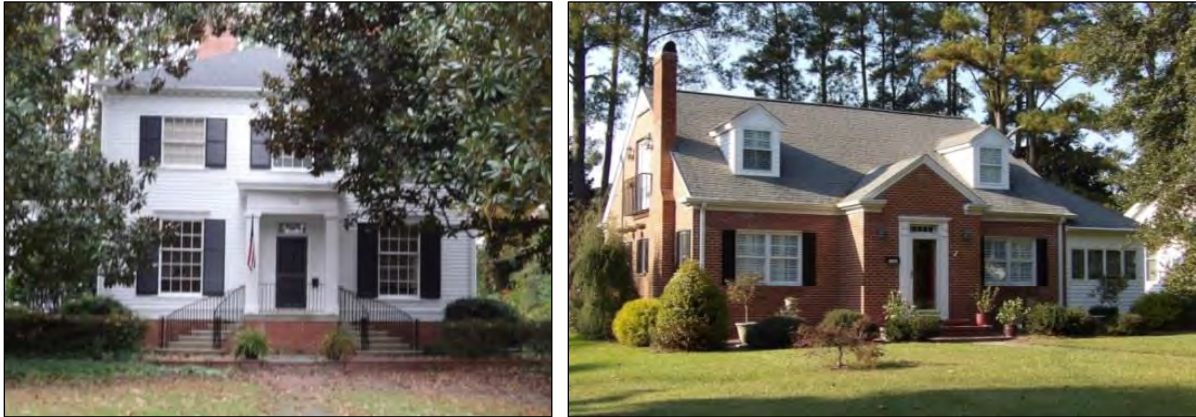
Photo 20: Examples of Georgian Revival (1102 Summit Avenue, Left) and Colonial Revival (1202 N. Market Street, Right) Houses within the North Market Street Historic District.
