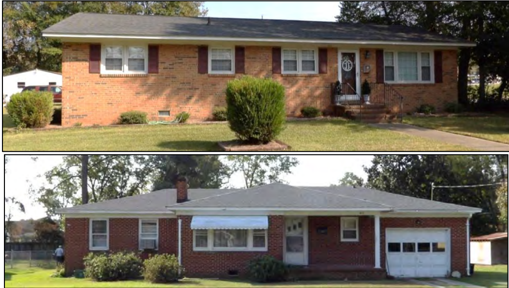
Photo 62: Ranch-Style Houses at 428 E. 12 th Street (Top) and 417 E. 12 th Street (Bottom)
