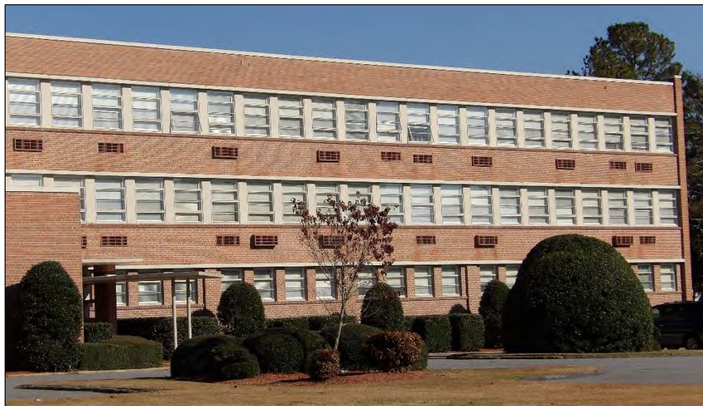
Photo 51: Window Detail, Southwest Elevation, Bertie Memorial Hospital (BR0344).
