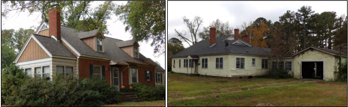
Photo 69: Houses 301 W. 15th Street (Left) and 209 W. 15th Street (Right).
