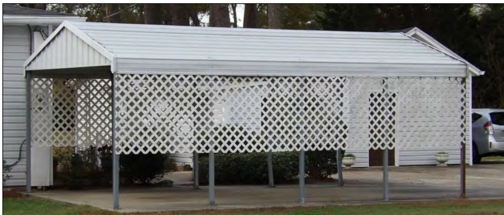
Photo 5: Carport, North Oblique.
