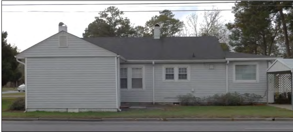
Photo 4: House at 1498 N. Market Street, Northeast Elevation.
