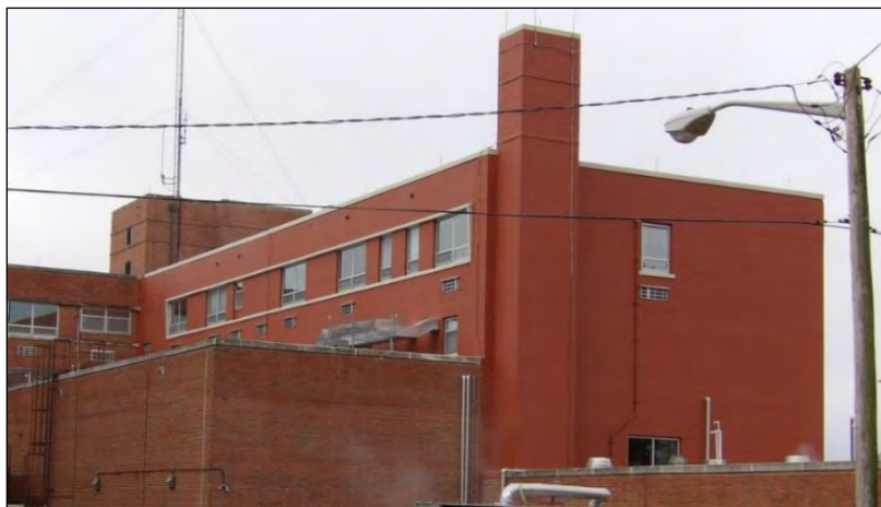
Photo 34: Northeast Oblique of the Original Rear Ell.
