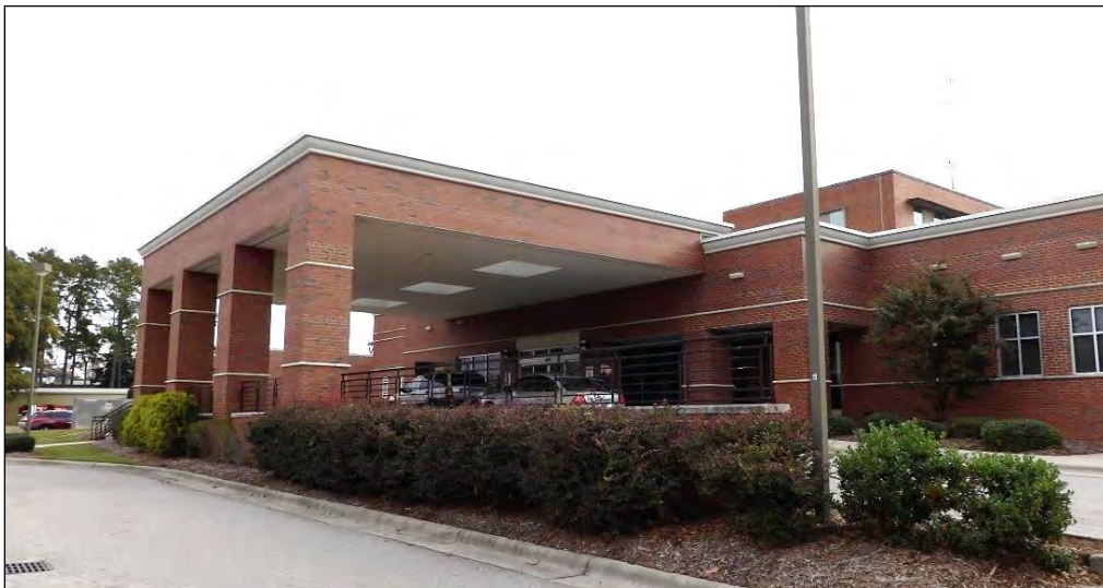
Photo 45: Modern Porte-Cochère Extending from the West Elevation of the 2008 Addition.
