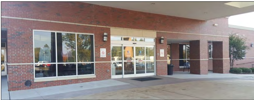
Photo 44: Current Primary Entrance Located on the 2008 Addition's West Elevation.
