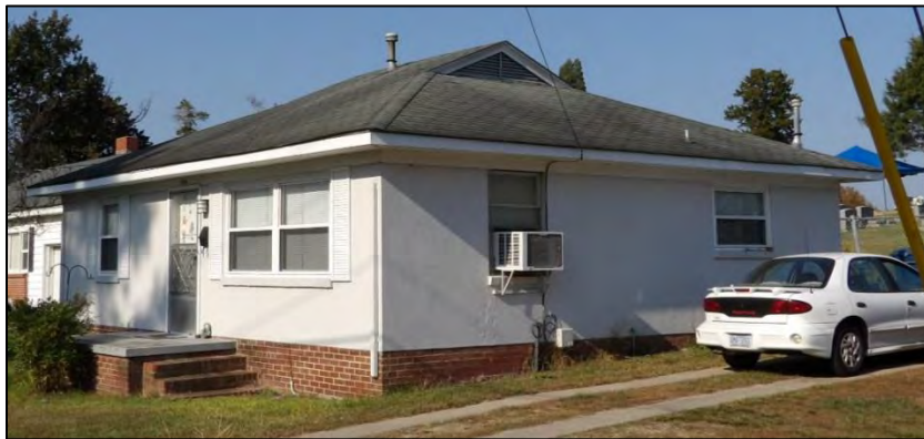
Photo 56: 304 E. 15 th Street. Note the replacement vinyl windows.
