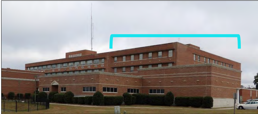
Photo 36: Southeast Oblique of Vidant Beaufort Hospital; Eastern Wing Noted in Light Blue.
