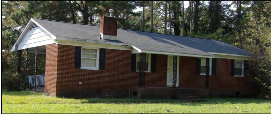
Photo 71: House at 307 W. 16th Street, example of a side-gabled roof with an interior-front brick chimney.
