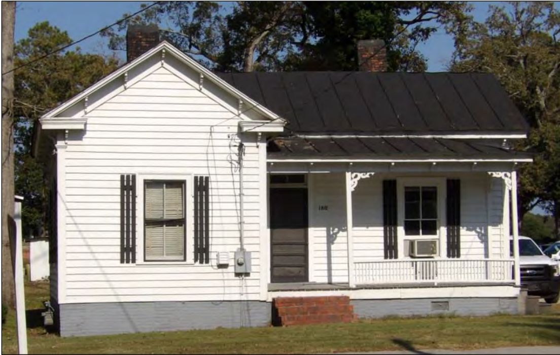
Photo 14: Caretaker's Cottage, Southwest Elevation.
