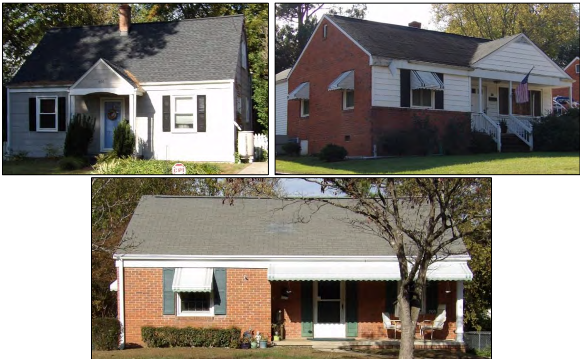
Photo 66: Examples of Dwellings within the Hi-Mount Historic District (WA4512): 605 Mills Street (Top Left), 712 Mills Street (Top Right), and 709 Mills Street (Bottom).
