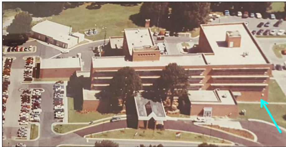
Photo 35: 1989 Photograph Showing the Eastern Wing. 90
