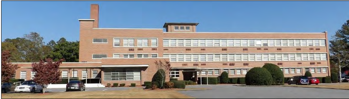
Photo 50: Bertie Memorial Hospital (BR0344), Southwest Elevation.
