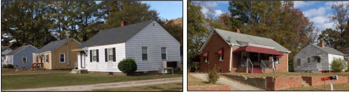
Photo 65: 800 Block of Leggett Road (Left) and 836 Ellison Drive (Right) in Lincoln Park Historic District (ED1555).
